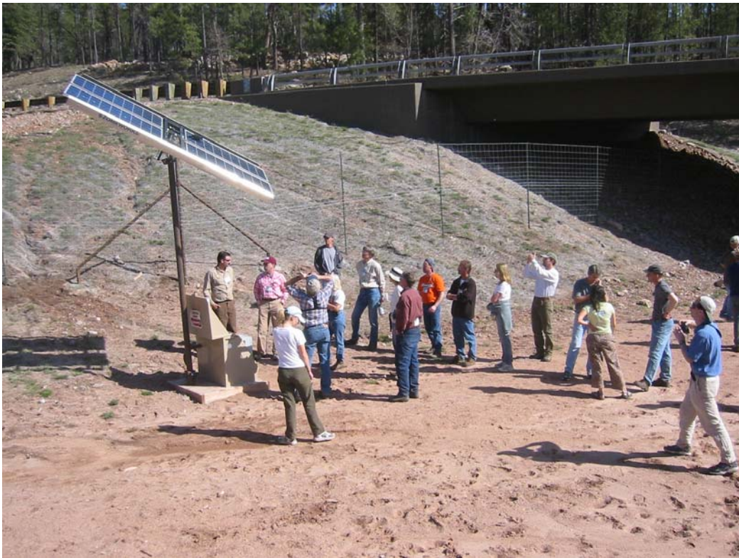
Video equipment is powered using solar panels to monitor species using the underpass.
