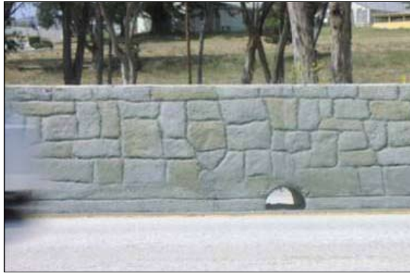
Median barrier on Highway 1 near San Luis Obispo, California, with openings for small animal passage.
